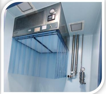
Performance: Air Cleanliness- ISO Class 5 [ISO 14644-1:1999 (E)]; Air Velocity- 0.45 ± 0.05 Mps.
