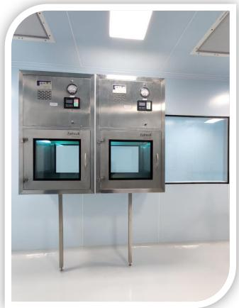
Performance: Air Cleanliness- ISO Class 5 [ISO 14644-1:1999 (E)]; Air Velocity- 0.45 ± 0.05 Mps.
